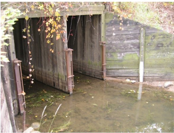
Upstream side of Carlson Bridge
