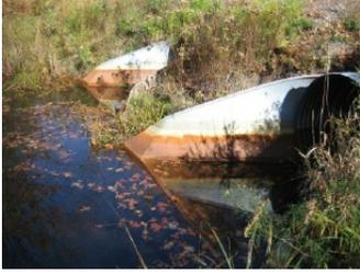
**Culverts downstream side of NN with standing water from backup caused by 7+ beaver dams downstream.**
