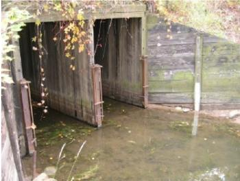
**No stop logs on 09/26/2006 despite low water level on Round Lake system.**
