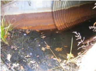
**The culverts on NN are almost dry on 10/10/2006. Note higher level water staining.**
